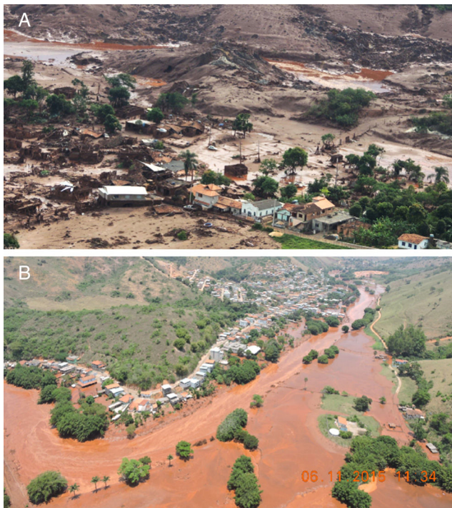
Fig. 3. Buildings affected by the Fundão tailings dam: (A) District of Bento Rodrigues, Mariana and (B) Urban area of the municipality of Barra Longa.
