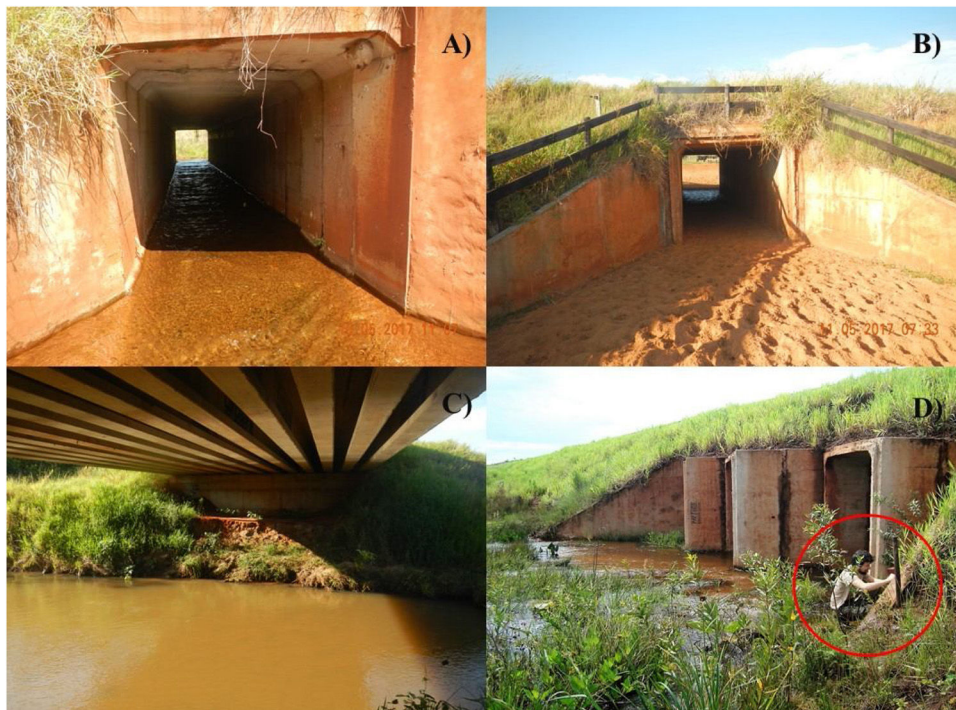
Fig. 2. Types of underpasses monitored along Highway MS-040 in Mato Grosso do Sul State, Brazil: (a) drainage culvert, (b) cattle box, (c) bridge and (d) view of drainage culvert, red circle shows the installation of the camera-trap outside of the structure.
